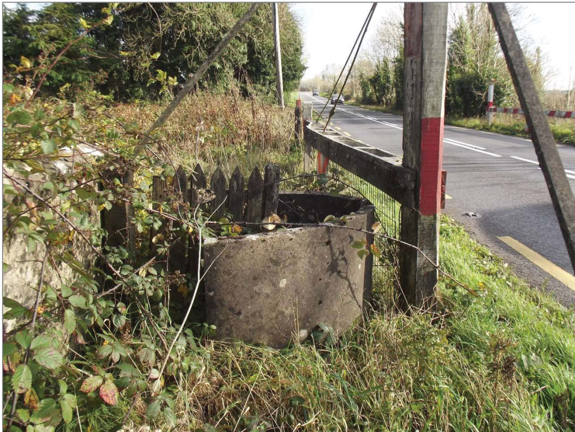
Illus. 5.7 and 5.8—Railway crossing on the N17 (Inventory No. 7). Options 1 and 2 would affect the boundary wall and pedestrian stile (below); Option 2A would result in the demolition of the keeper's cottage also, which is rated a severe impact of the road project.
